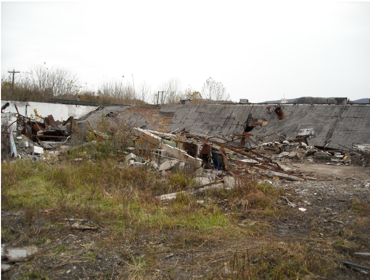
View of Collapsed portion of main building where asbestos was released into the environment. Taken November 2010.
