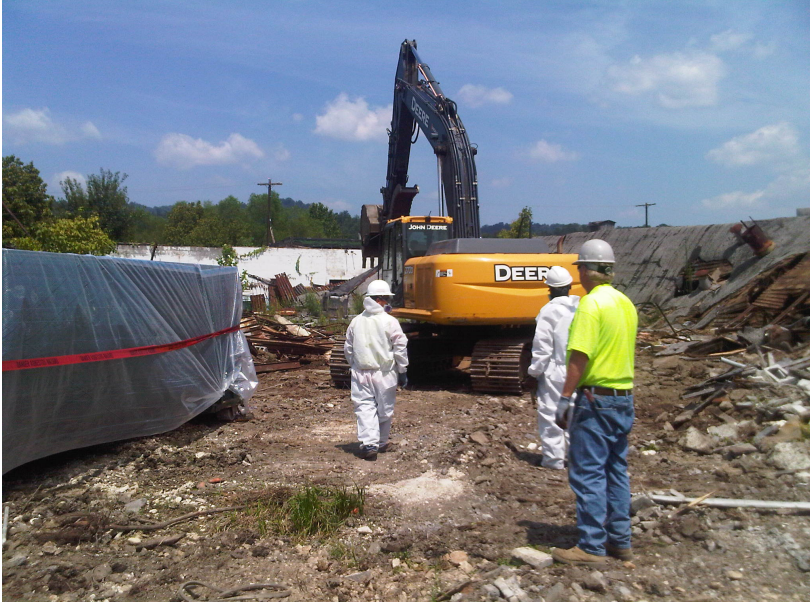
Building demolition and asbestos removal, Fall 2011.
