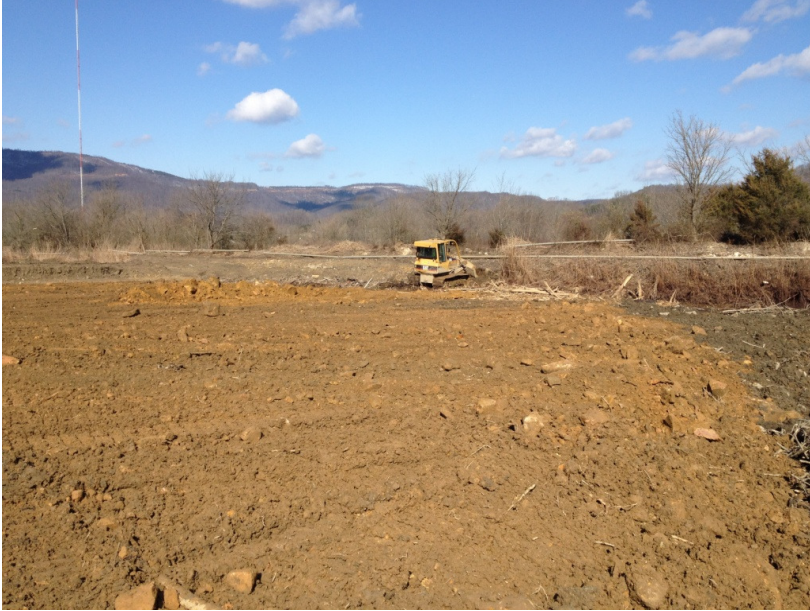
Filling and capping sediment ponds. Late winter, 2012.
